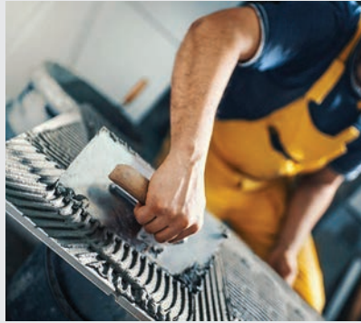
GLUING THE SLAB
