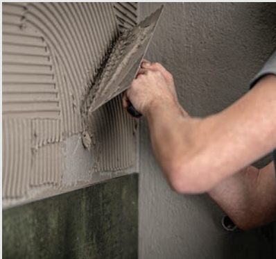
GLUING THE SUPPORT
