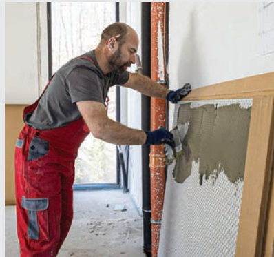
GLUING THE SLAB
